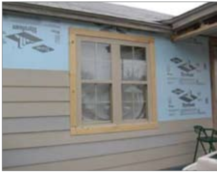
New siding installed on Mr. and Mrs. C's home.
